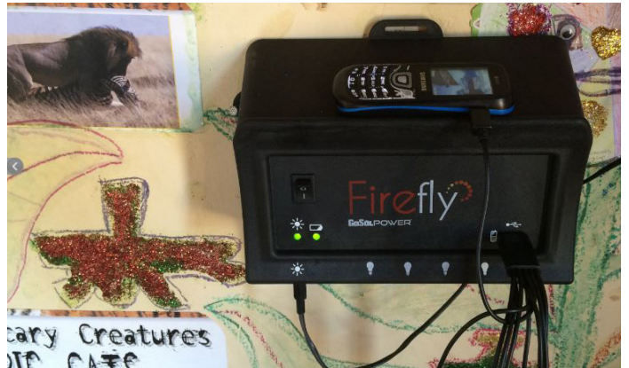
The controller for a Firefly solar-powered lighting system installed on a wall in Tanzania.
